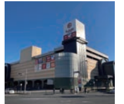
A commercial facility (in the Tokyo metropolitan area)
