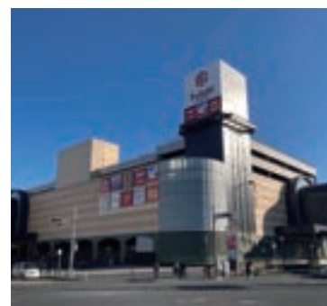
A commercial facility (in the Tokyo metropolitan area)
